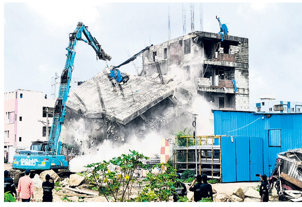
An excavator being used to demolish an illegal building in Hyderabad
