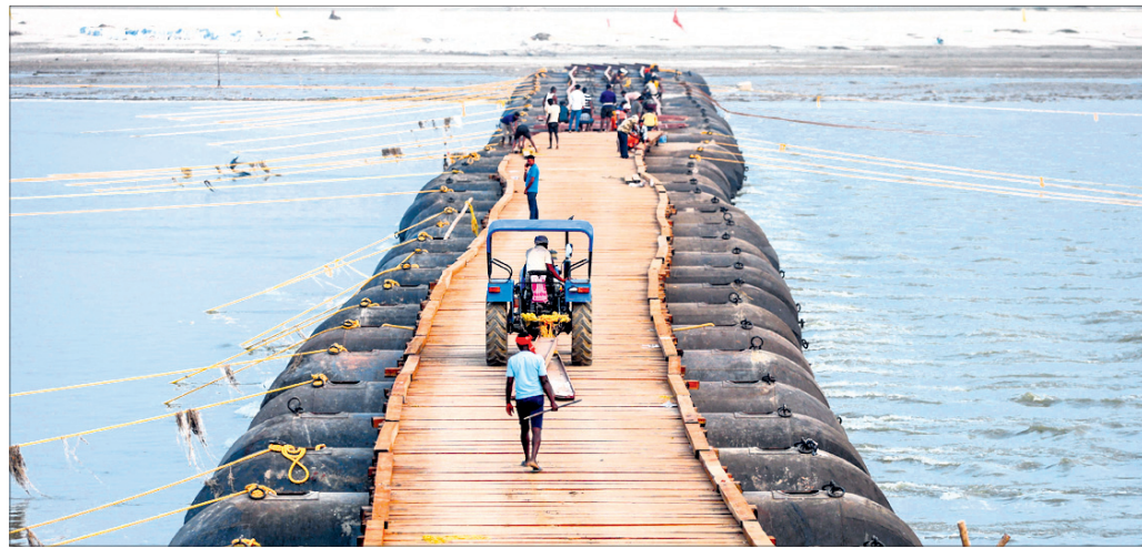
A pontoon bridge being made ahead of the 'Maha Kumbh Mela', at the Sangam, the confluence of three rivers the Ganga, Yamuna and mythical Saraswati in Prayagraj, Uttar Pradesh
